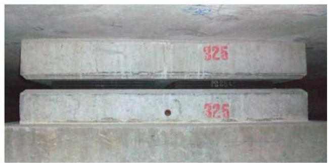
Figure 8. Photos of earthquake-resistant bearing pads and their reinforced-concrete support blocks.
